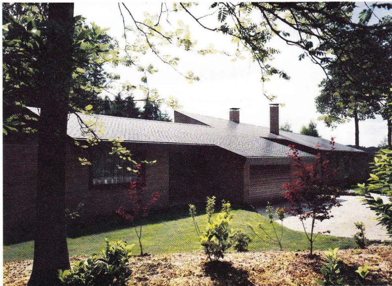
Asbestos cement shingles used in roofing.
