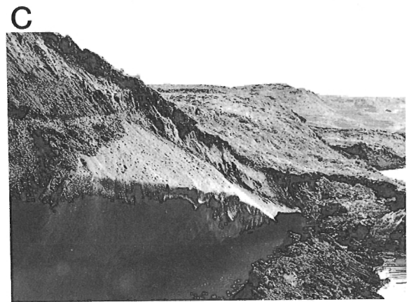
Figure 5. Site 3 at Hot Weather Creek: (a) low level oblique view of the retrogressive thaw slump, note the outline of a former structure marked by a dashed line, (b) massive ice unit exposed in the main bowl of the slump, location marked "b" in Figure 5a, and (c) an oblique section of an ice wedge exposed in stream bank.
