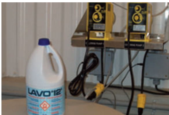
In-line chlorinator and concentrated bleach
