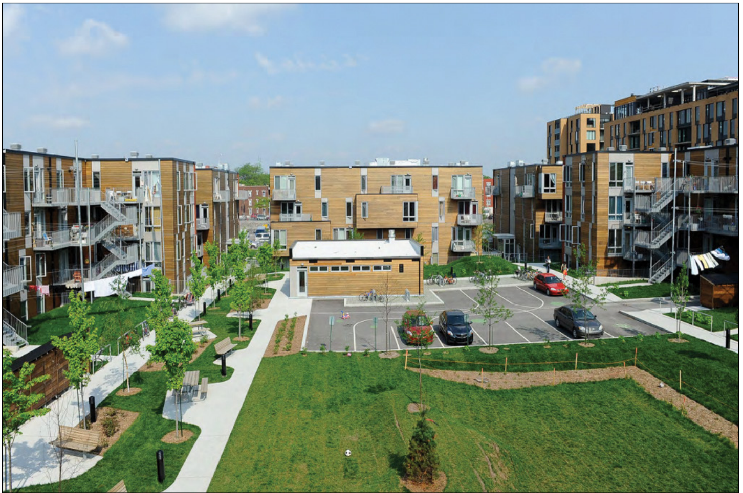
Figure 10 Stormwater retention basin in bottom right-hand corner (Credit: Nikkol Rot)
