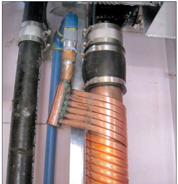
Figure 7 Drainwater heat recovery unit (Credit: L'OEUF s.e.n.c.)
