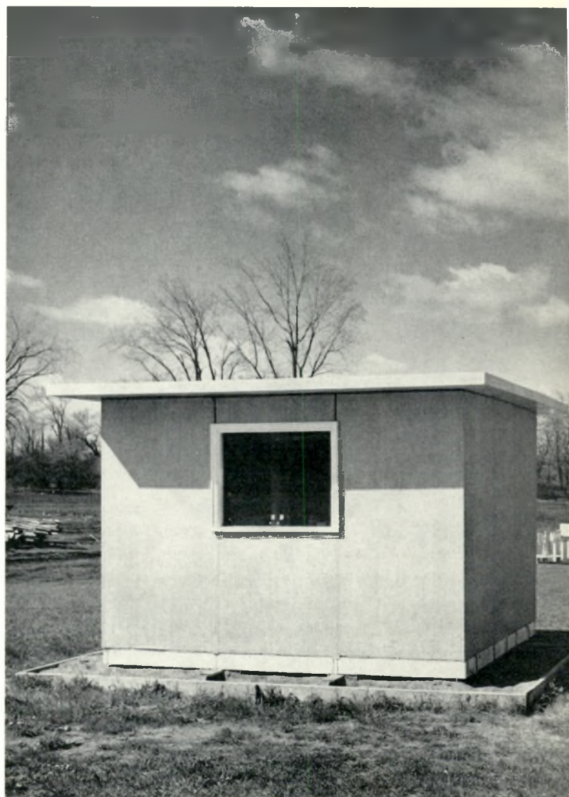
The foamed plastic hut erected on the grounds of the National Research Council, Ottawa.
