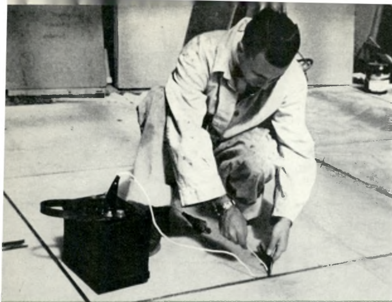
Fusing the plastic pipes, which are embedded in the substance of the floor, during the erection of the foamed plastic hut.
