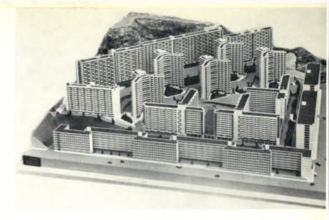
is being explored for the Ma Tau Wai project mentioned above. Piling is usually required for foundations, whilst at So Uk, for some point blocks, soil stabilization has been carried out. Finishings are kept extremely simple and considerations of overall proportion and site planning therefore become of tremendous importance.
