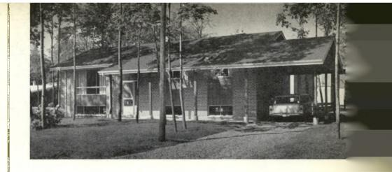
To this standard plan have been added certain characteristics that have resulted in a distinguished and interesting house. By raising the floor level three steps above grade, good natural light is achieved in the basement and the service entrance is direct and allows access to the bathroom from the basement.
