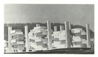
SYSTEM C Unlike systems A and B, system C is primarily "walk-up" accommodations, although the system also uses up to twelve storeys in height. Individual central cores lead to the dwellings.
