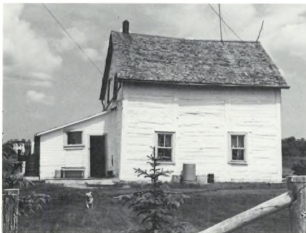
Fisherman's house in Selkirk, Manitoba showing the poteaux sur sole form of construction (also known as the Hudson's Bay or Red River Style).
