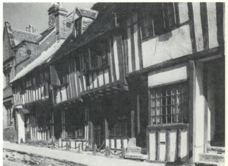
Tudor houses, Hastings, Sussex, England used a heavy timber frame with exterior infilling of wattle and daub. Such were the first English houses built in North America. Photo: U.K. Central Office of Information.
