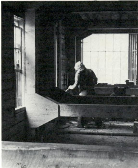
The walls were supported with interior bracing before the building was moved.
