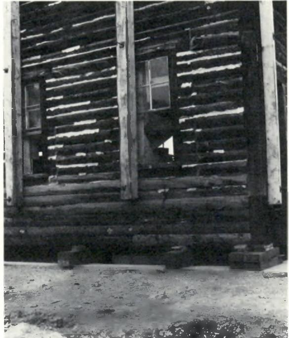
October 1977: the building was moved from the site, new concrete foundation pads were laid, and it was jacked back into position.
