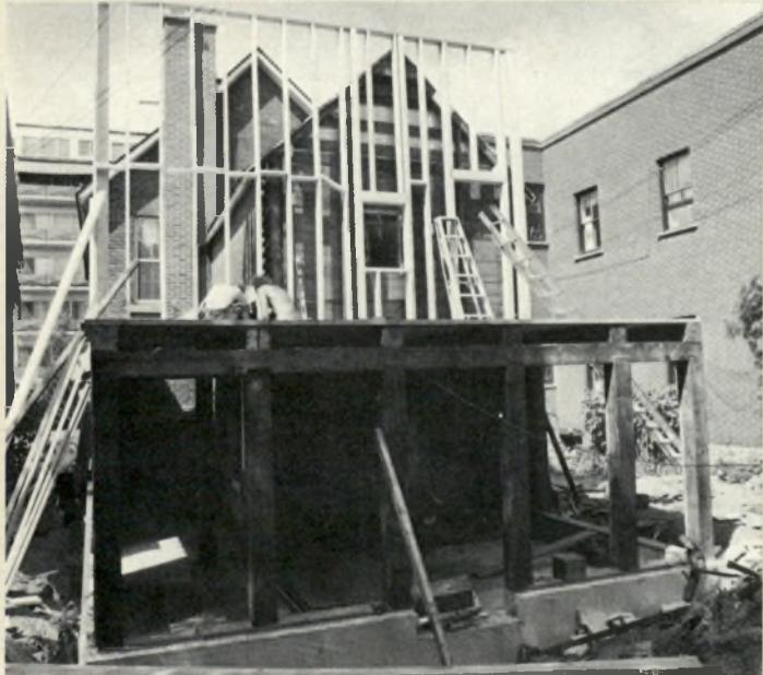
**2** The end wall has been dismantled for addition of a post and beam structure below. Brick removed from the exterior will be recycled into an interior thermal storage wall in the downstairs room.
