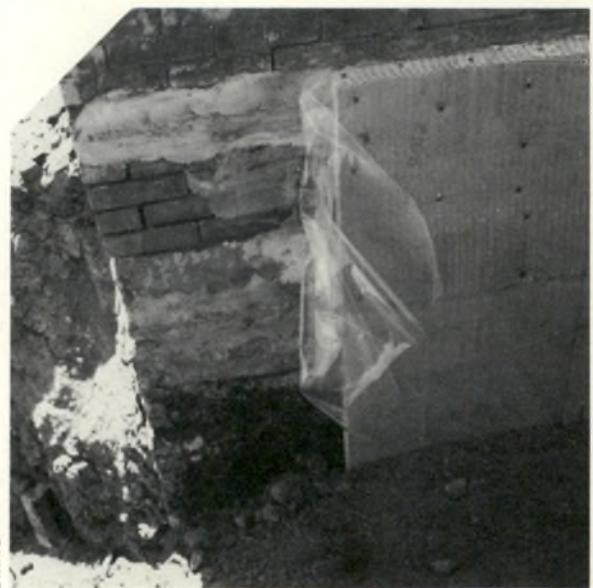
**Black foundation coating at bottom, level parging at top to hold glue for insulation. At right: insulation applied to a depth of 1200 mm, covered by polyethylene vapour barrier and metal lath in preparation for parging above grade.**
