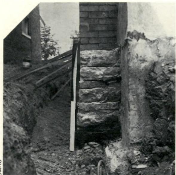
This view shows dead air space behind the insulation, sealed at the top by glue and parging. Black foundation coat can be seen at bottom.
