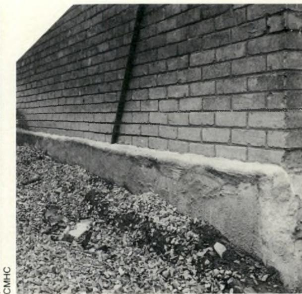
Job completed, except for metal flashing yet to be applied to protect the join between wall and foundation.
