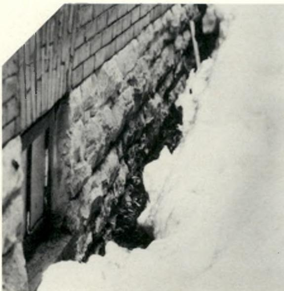
**The problem:** In winter, heat escaping through the stone melts the snow. Freezing and thawing loosens mortar, allows seepage during the spring, and creates dampness whenever there is moisture in the ground.
