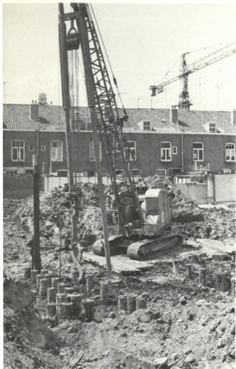
After structural demolition, old wooden pilings must be pulled like decayed teeth. New pilings will be tubes, filled with concrete after they are sunk.
