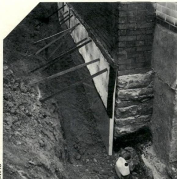
Insulation glued to parging and covered with metal lath is propped up while glue hardens. Container of concrete weld to be mixed with mortar mix for exterior parging is at lower right.
