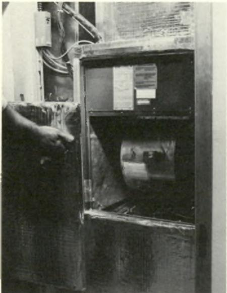
Indoors: heat pump unit specially insulated for the NRC trials.
