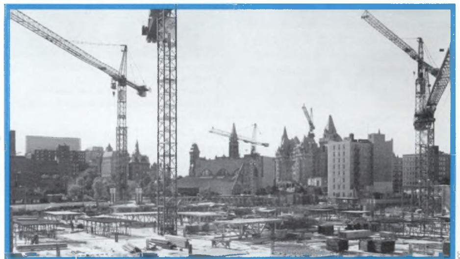
*The Rideau Centre shopping mall took 21 months to construct. During the building period, an average of 1 000 construction workers were on-site every day. The site was originally the turning basin for barges at the northern terminus of the Rideau Canal. Some 181 000 t (metric tons) of stone were needed to provide a solid foundation for the Rideau Centre complex.*
