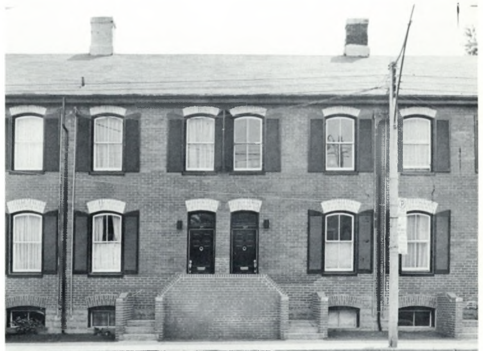
Rehabilitated row housing in central Toronto in the general area of the Trefann Court urban renewal project.
