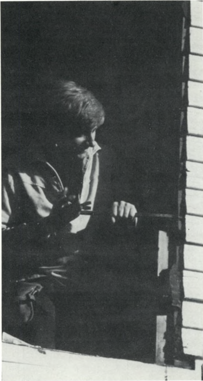
A rough opening is prepared for a new window.
