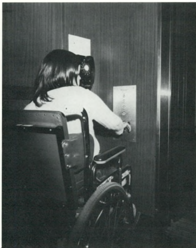
The control panel in the elevator can easily be reached from a wheelchair.
