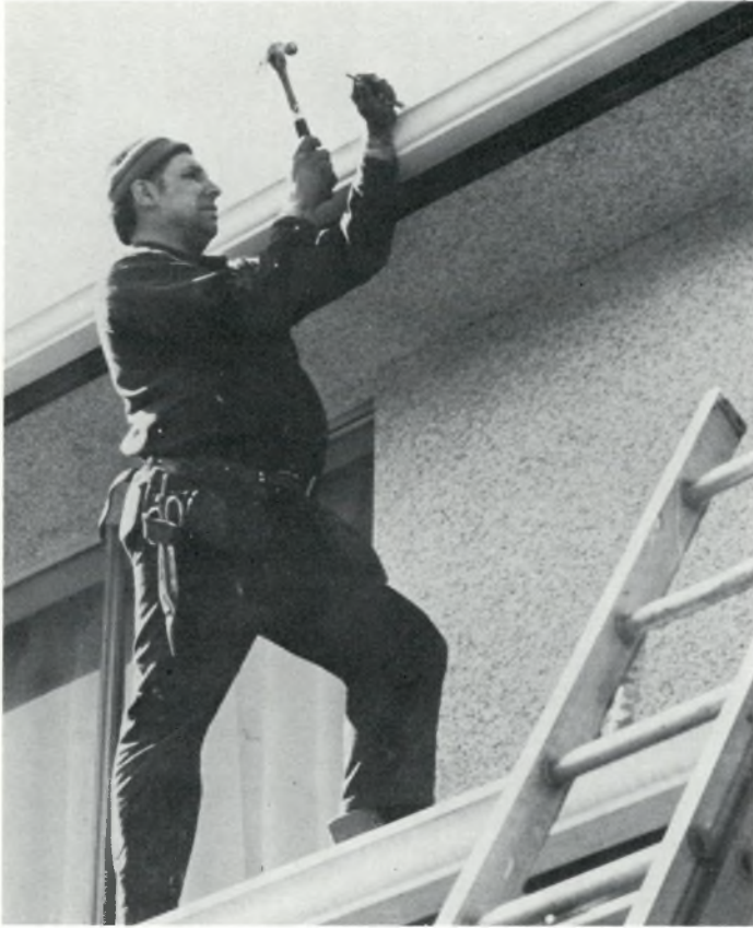
A new eavestrough is installed.
