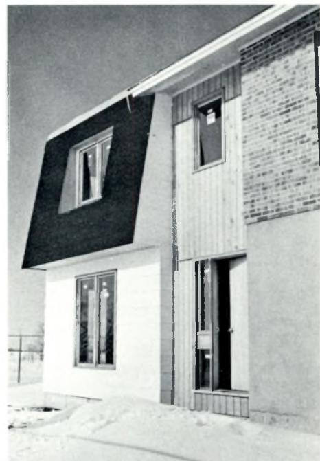
This test building at Uplands Airport, Ottawa, is the result of collaboration between Central Mortgage and Housing Corporation, National Research Council and the Ministry of Transport. Experiments are being carried out to gather data on forms of construction which can reduce aircraft noise within individual dwellings.
