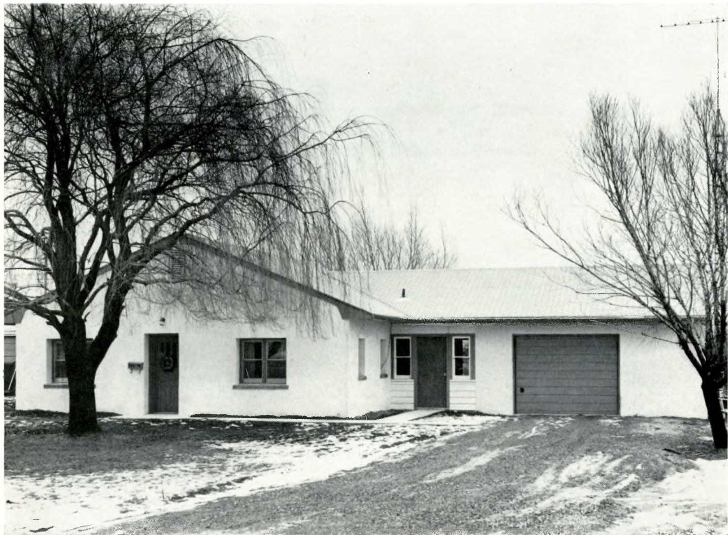
With rehabilitation work complete, home has new exterior wall finish, a gable roof and an attached two-car garage. Lot was regraded to improve setting and cure drainage problems. Owners throughout urban renewal area are now applying to CMHC for similar loans to modernize and rehabilitate their properties.
