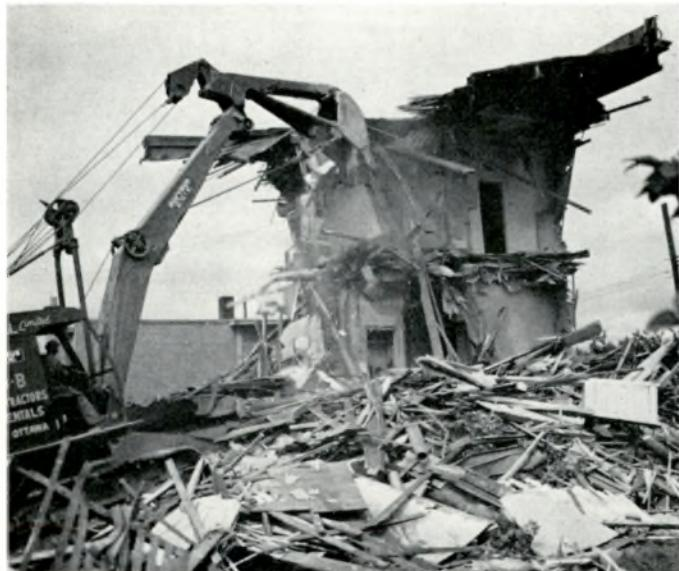
Demolition in Ottawa's Preston Street Urban Renewal Project as contractor moves in on core of three-storey, wood-frame building. The structure was originally built to house an early Ottawa school, subsequently converted to a six-unit apartment building.
