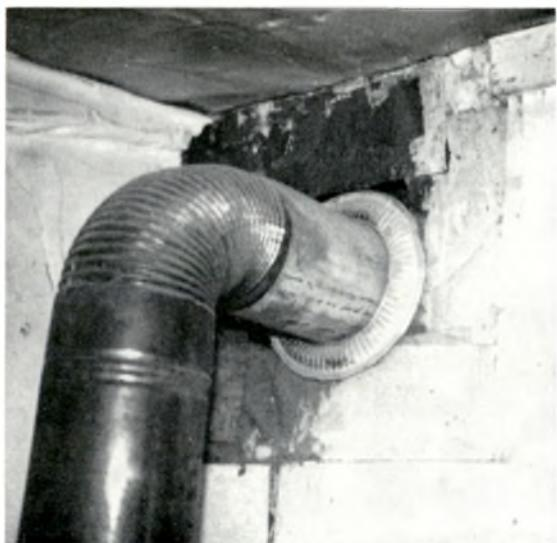
Stove pipe from range. Note poor entrance to chimney and seepage of tar.
