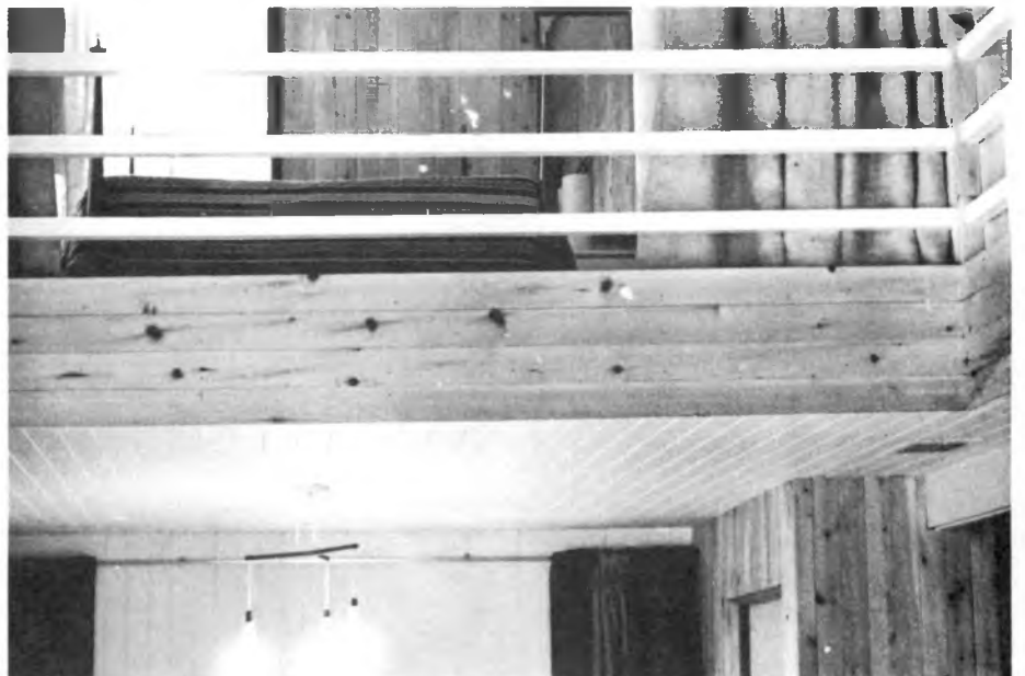
The open balcony above the two-storey living room.
