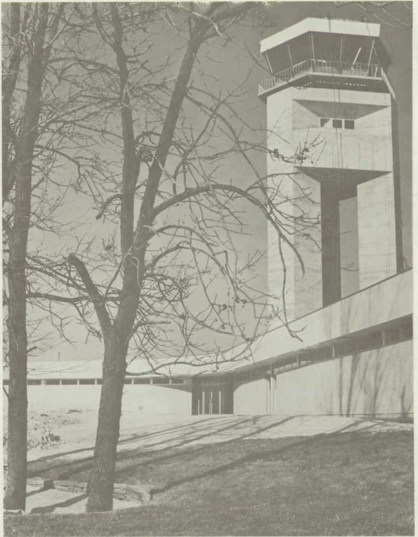
This three-legged traffic control tower forms part of the complex air traffic control facilities at Toronto International Airport.
