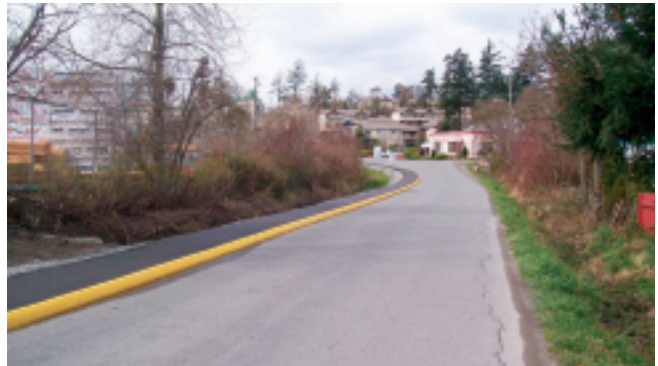
Songhees Nation also used tax revenue for road paving, sidewalks, a drainage upgrade system and a playground.
