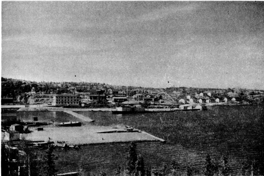
5. The residential area at the Giant mine is smaller, more compact and more recent than the one at Con. All but one of the single-family houses are contained in this view. The large white building left of center is the residence for single staff employees.
