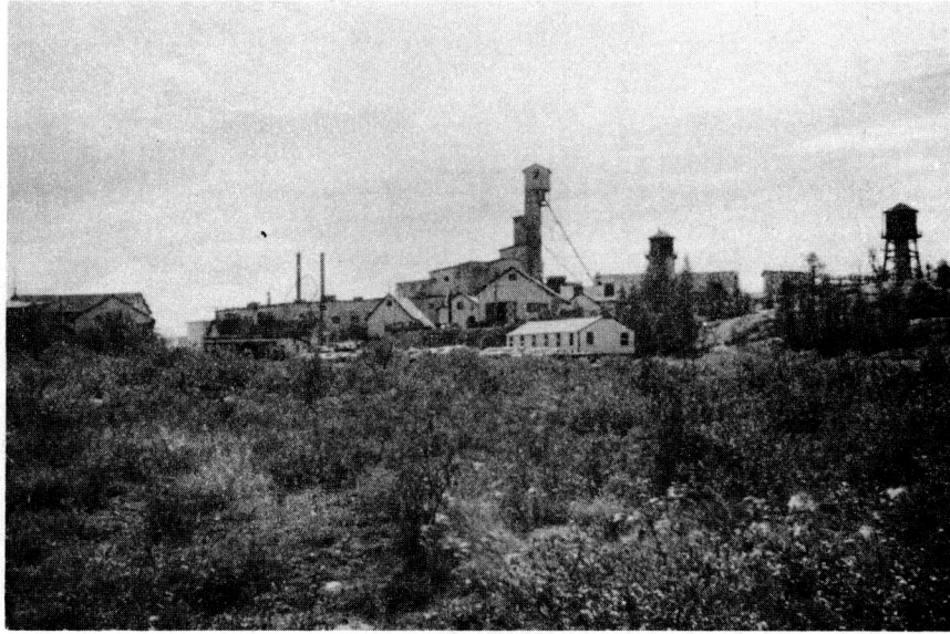
18. By far the most prominent features of the local landscape are the headframes and mine complexes of Giant and Con. This illustration shows the active headframe of the Con-Rycon mine.
