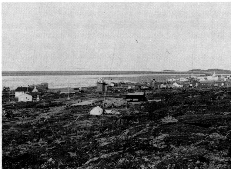
View of Coppermine from west, early June, 1963.
