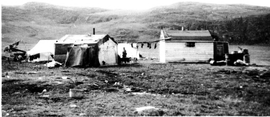
HOUSING BUILT FROM SCRAP LUMBER
