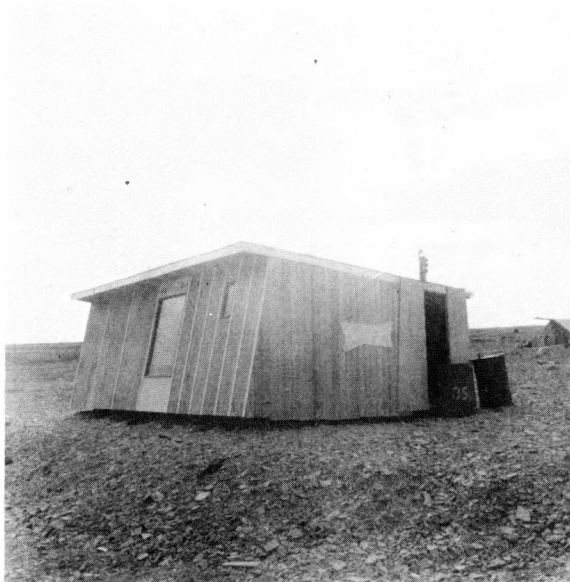
PLATE 17 – One-bedroom house, type built 1965-66 (photo K. Crowe)
