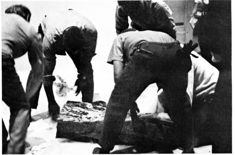
First stone of inukshuk about to be hoisted into position
