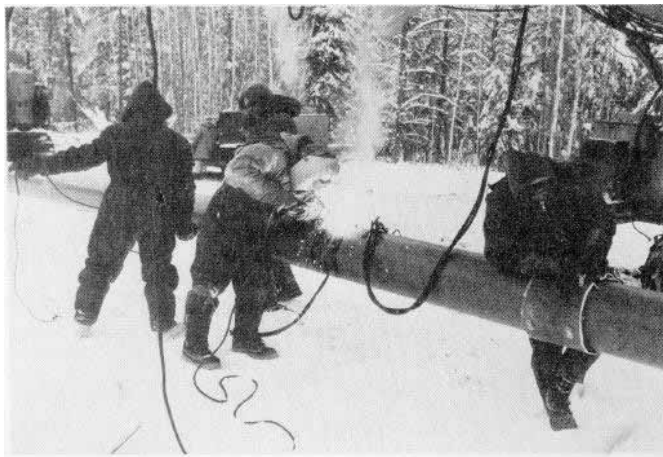
Welding together two sections of pipe.
