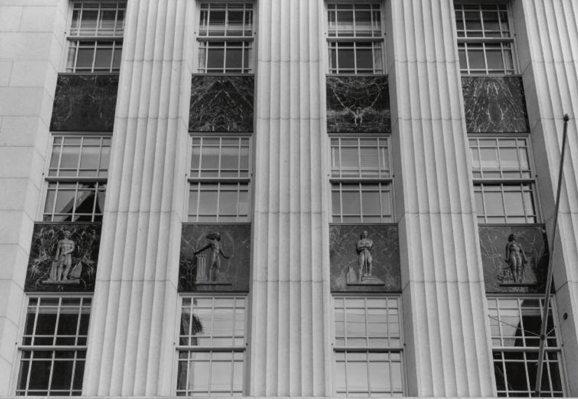
Detail of front facade. Between the windows are panels of polished Vermont Verde Antique marble. Those in the lower row feature bronze allegorical figures by renowned Canadian sculptor Jacobine Jones.
