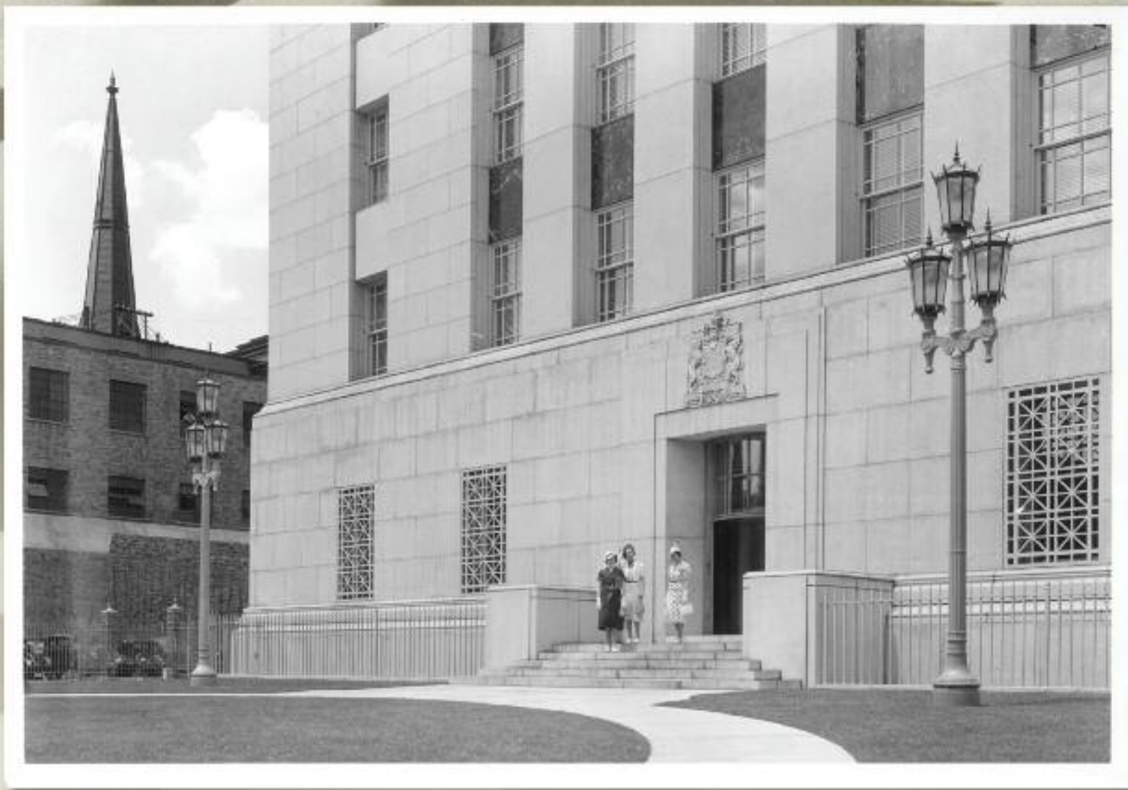
Sparks Street (south) entrance to the Ottawa Agency, ca. 1942. Flanking the entrance are ground-floor windows with protective grilles. The grilles were made of aluminum painted the same colour as the granite.
