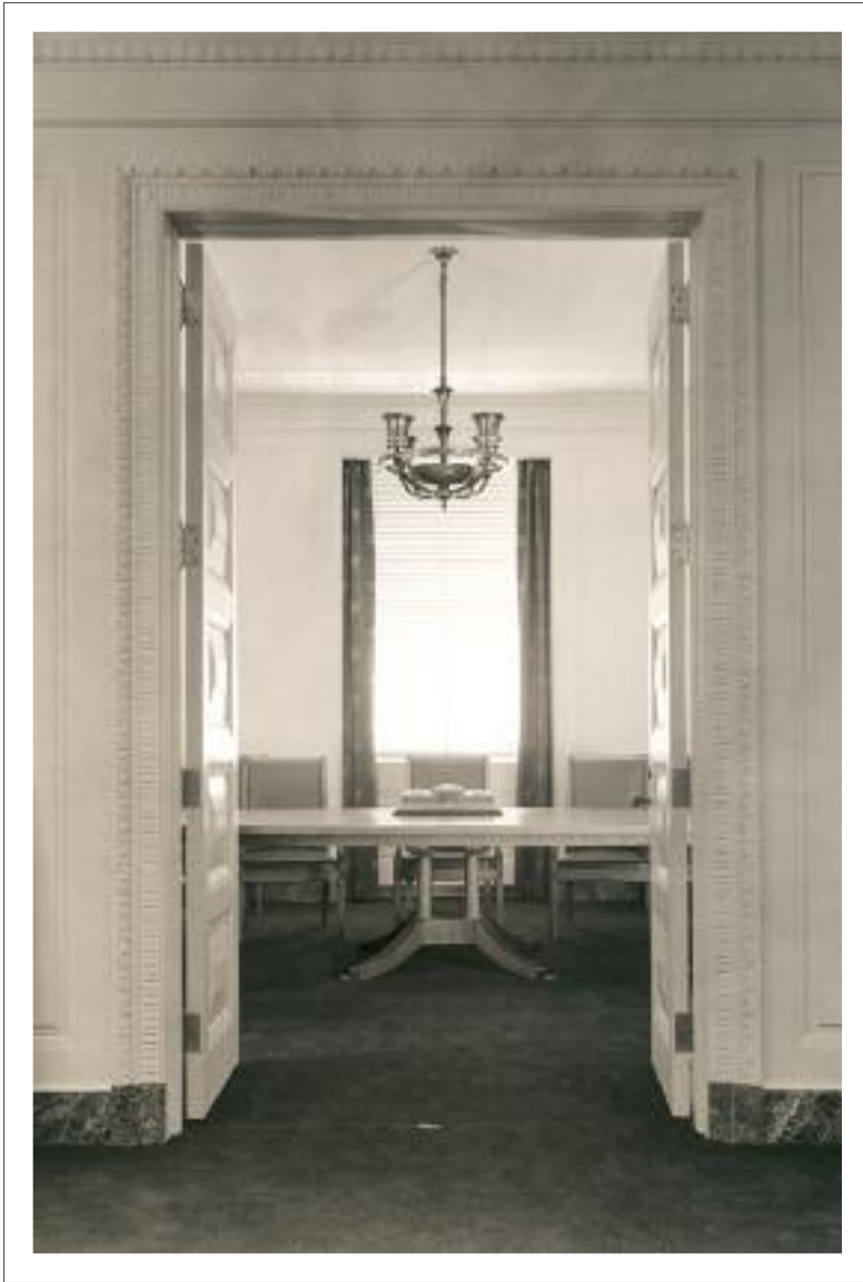
(Left) View of the Boardroom from the anteroom, 1938. Both rooms were panelled in cherrywood, painted a light putty colour, and were trimmed with a base moulding of Breche Portora Italian marble. (Right) Detail of moulding in Boardroom. Echoing the classical motif decorating the Sparks Street bronze doors, griffins and a Greek palmette guard the original Boardroom.
