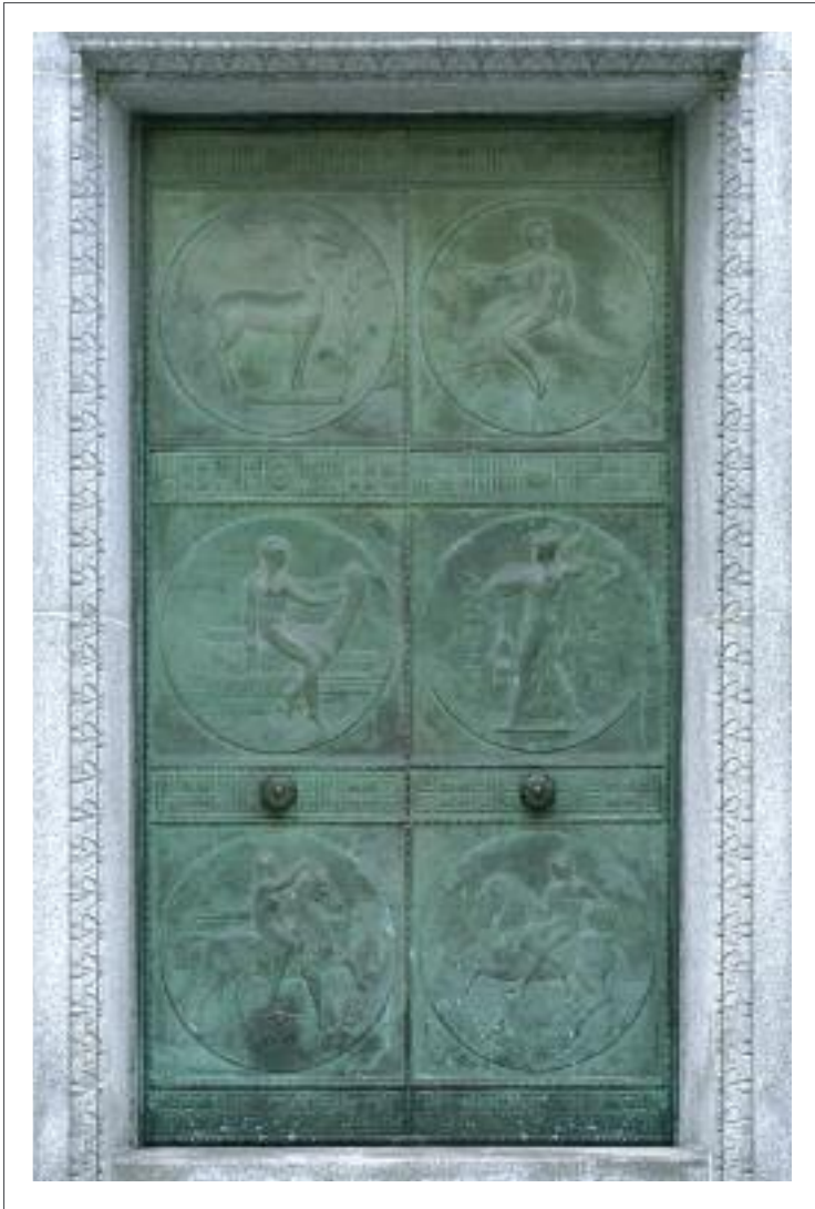
(Left) Bronze front doors designed by sculptor Ulysses Ricci of Ricci and Zari of New York and cast by the General Bronze Corporation of Long Island. In keeping with the building's classical theme, the doors feature Greek coins. The architects originally recommended a dragon motif, but the design was considered "too romantic." 7 (Right) Reverse of silver coin from the Greek city of Tarentum, Calabria, showing a man holding a cup while riding on a dolphin
