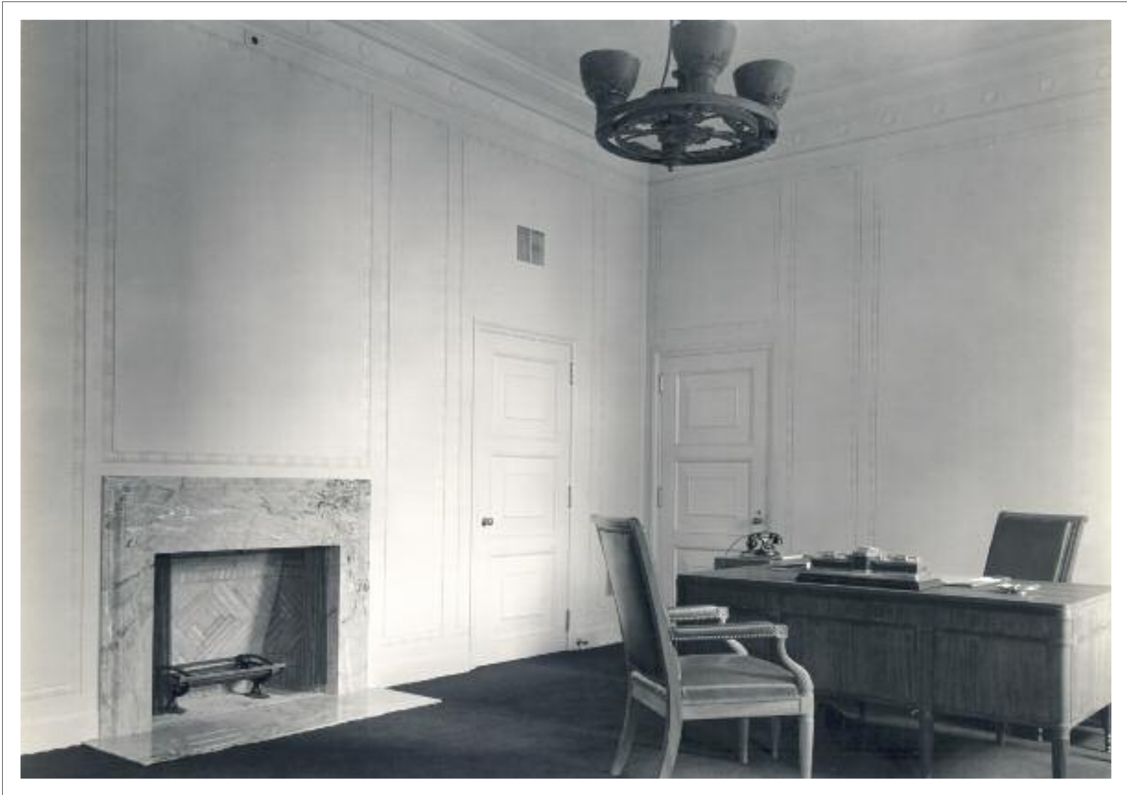
Office of the Governor, ca. 1938. Like the Boardroom, executive offices were panelled in cherry and painted a light putty colour. The Governor's office had a coal-burning fireplace with a hearth and surround of Loredo Chiaro Italian marble.
