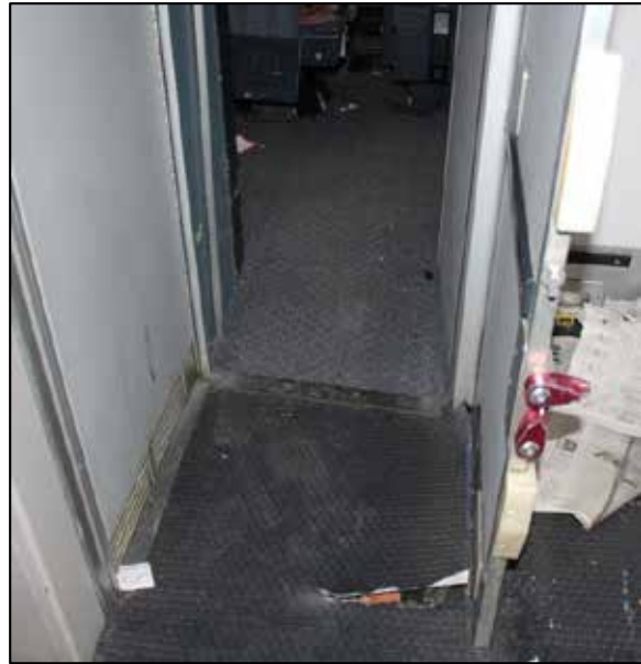
Figure 9. Floor damage aft of cockpit door
