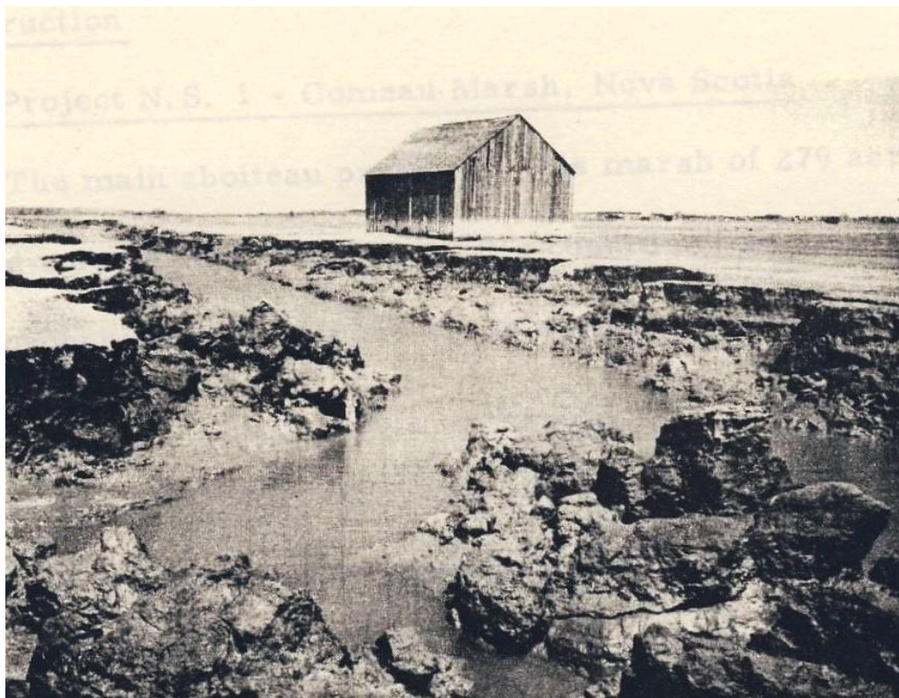
Figure 7: Marsh barn on the John Lusby Marsh National Wildlife Area circa 1949, after the dykes broke. Note the high-tide line partway up the outer walls of the barn (Dept. of Agriculture, Maritime Marshland Rehabilitation Branch, First Annual Report, 1950, page 10).
