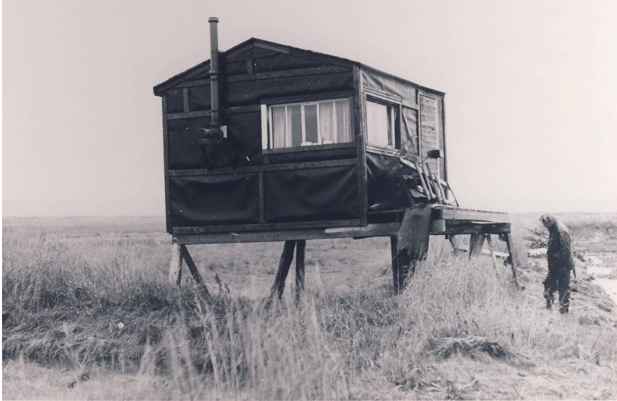
Figure 4: Old hunting cabin (no longer existing) at John Lusby Marsh National Wildlife Area, built on legs to allow higher tides to flow underneath
