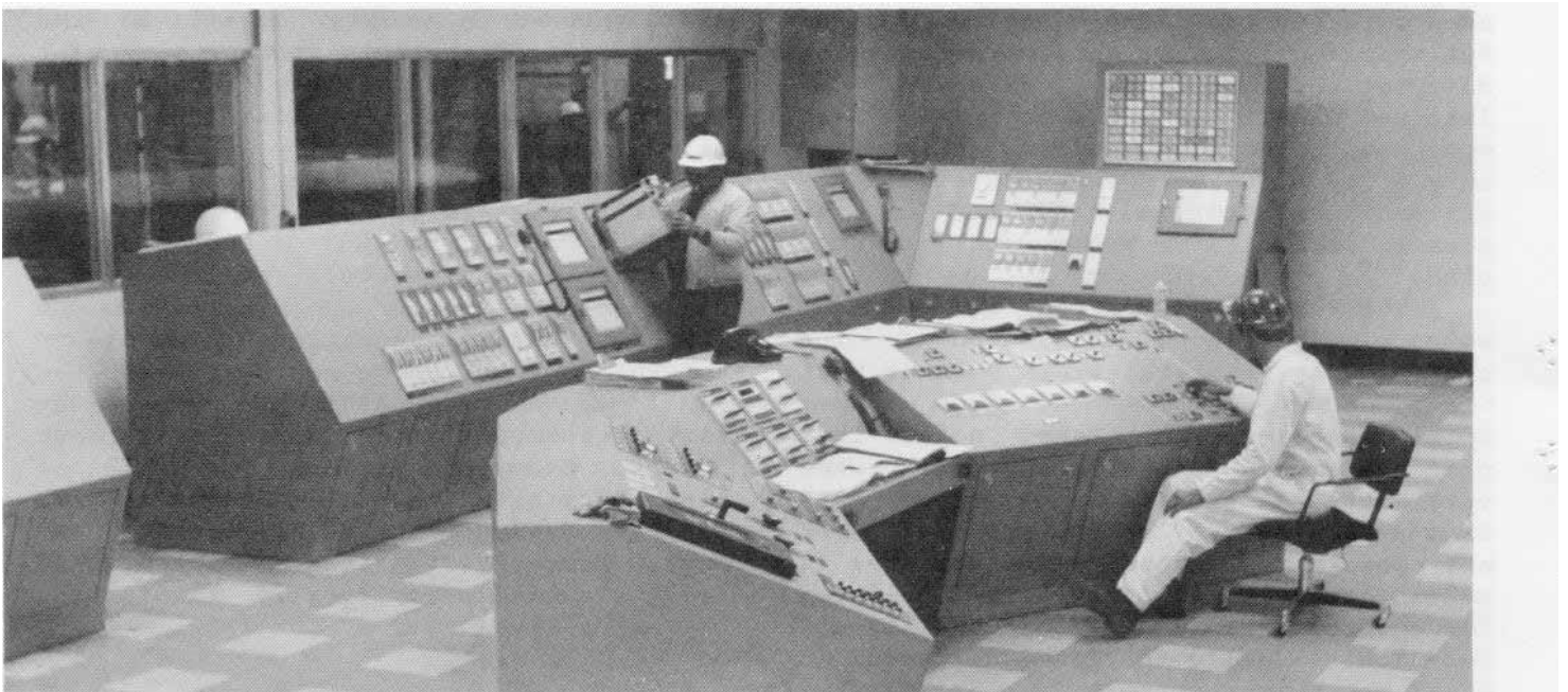
Eldorado's Port Hope UF 6 Refinery (Courtesy of Eldorado Nuclear Ltd.)
