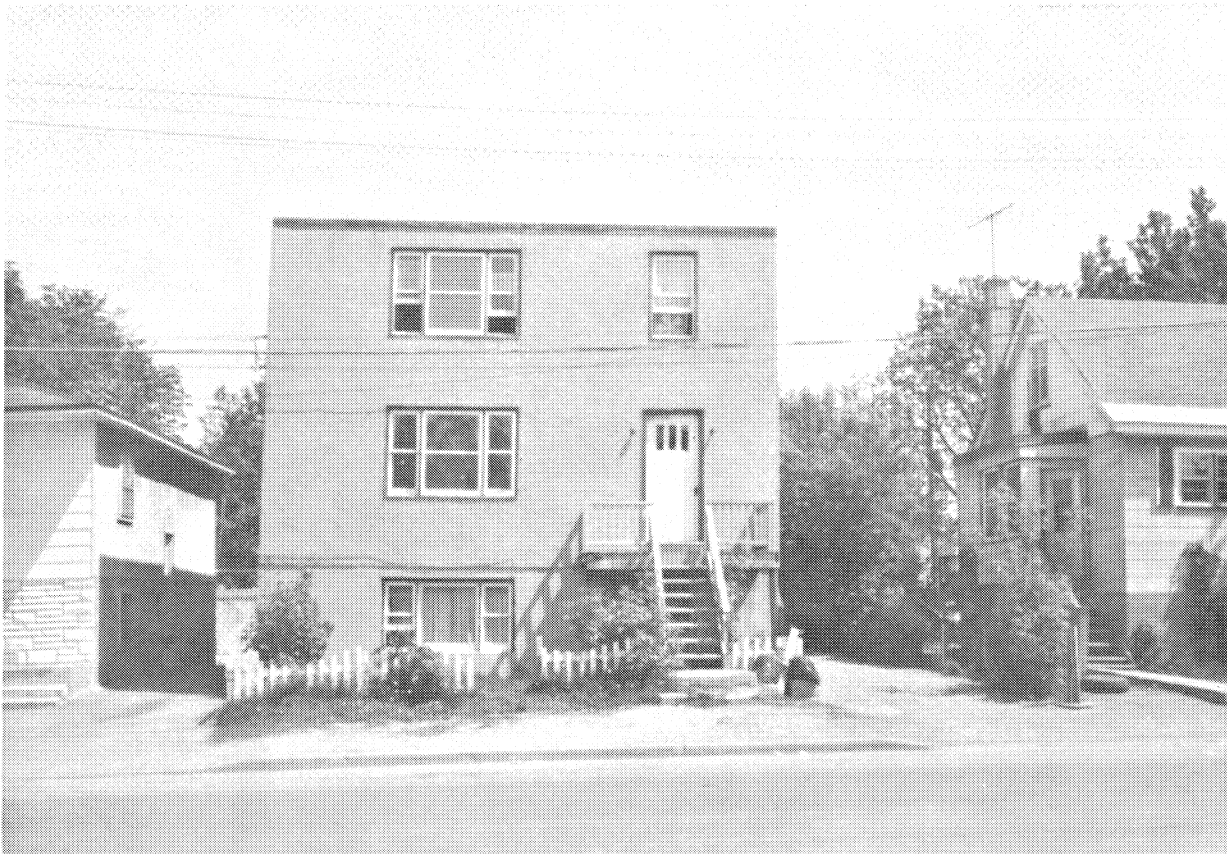
Figure 5: Apartment house, Vanier, Ontario. Building has settled 20 cm on one side.
