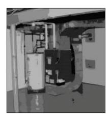
c. Make sure there are no partitions or articles, which might reduce air circulation, within 75cm (30") of the furnace. This is particularly important for gas furnaces which require the use of surrounding air for efficient combustion.
