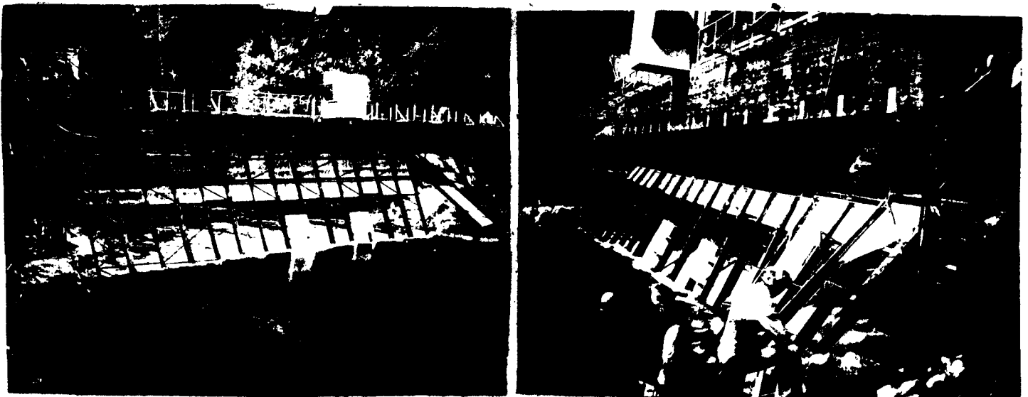
Initial lowering of frames for alignment with river bottom.
