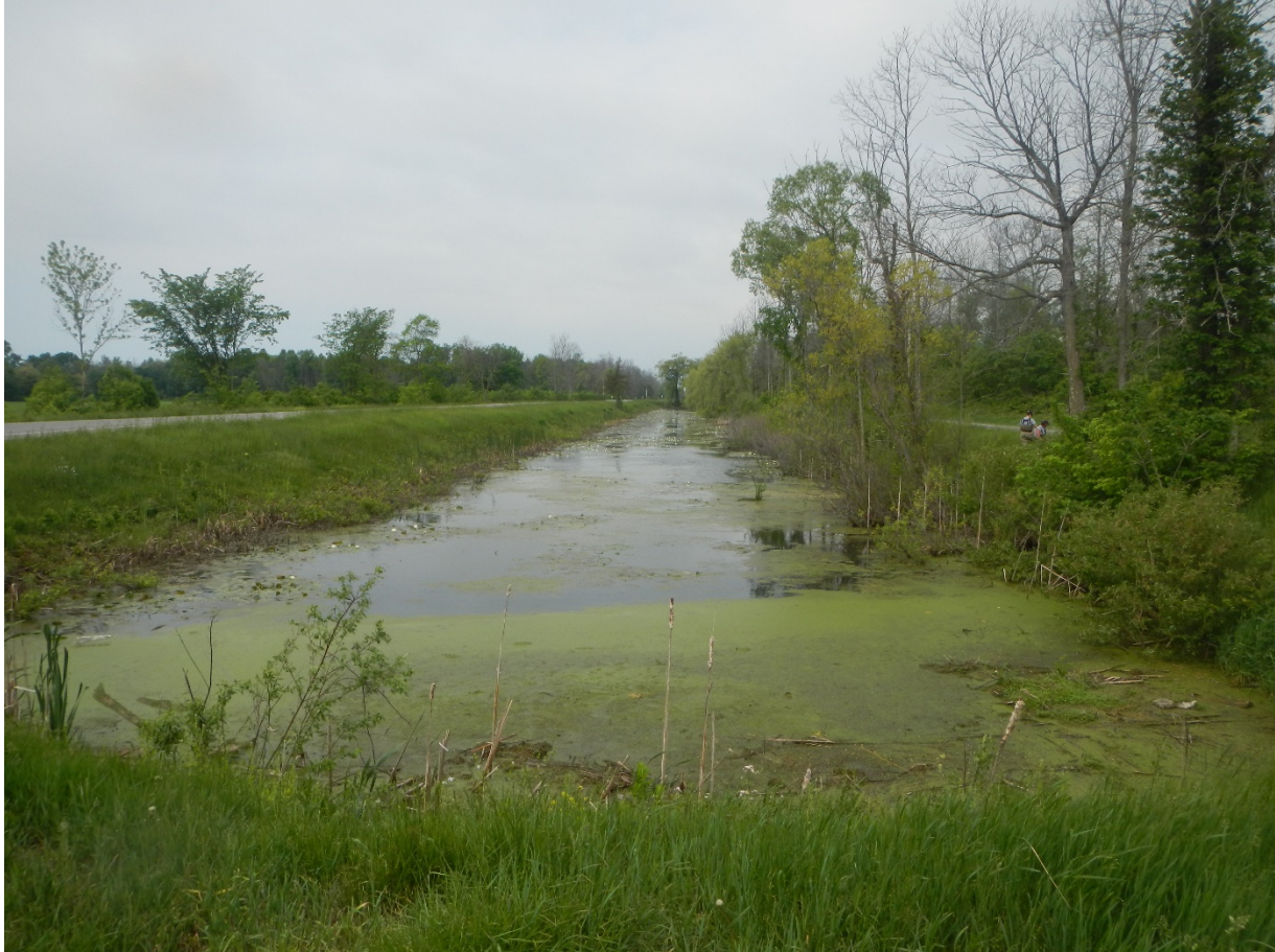
Figure 8. Site photograph of LON-FED-01 depicting the current state of stagnation and overgrowth which is consistent throughout the Feeder Canal.
