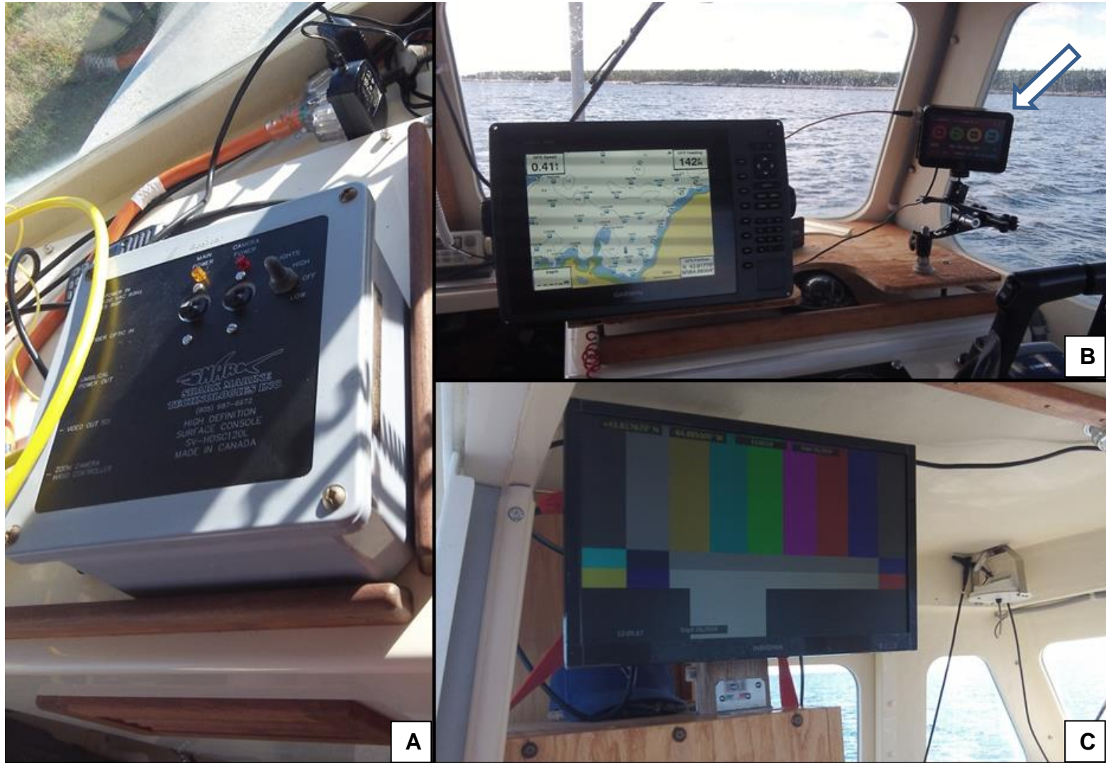
Figure 8: Electronics in wheelhouse. A – Camera control box; B – Garmin chart plotter with drop camera target points and Atomos HD recorder (arrow); C – LED TV.
