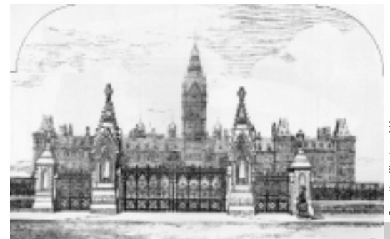
Wrought iron gates could be closed for security, 1876.
