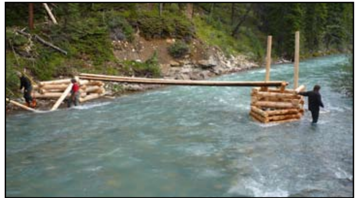
Trail Crew constructs a new bridge at Blue Creek, August 2008
