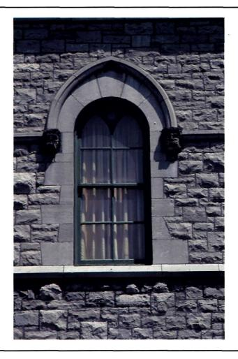
6 A typical upper storey window detail shows a range of stylistic influences: a Gothic Revival label moulding within which is set a window with a rounded Norman head, subdivided in an Italianate manner by wooden glazing bars. (Heritage Recording Services, Environment Canada — Parks)
