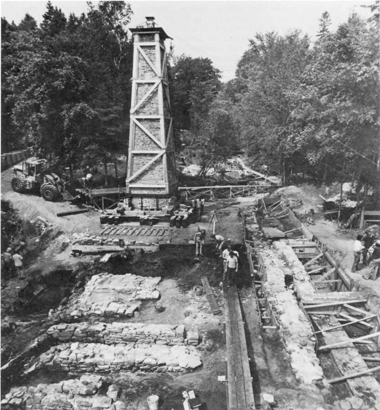
Archaeological excavations on the site of the lower forge. The refinery chimney was used to convert pig iron into iron. (Photo Parks Canada.)
