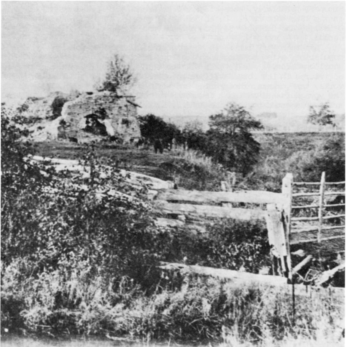
Ruins of the blast furnace ca. 1915. (Collection Louise Trottier.)
