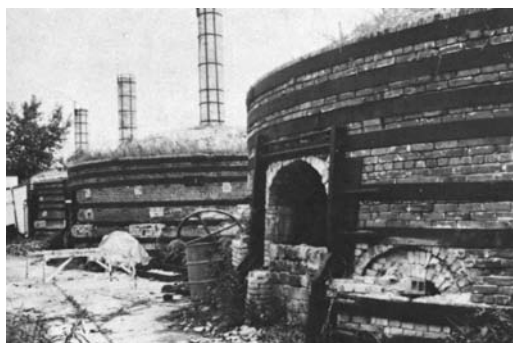
We are only beginning to appreciate monuments of industrial archaeology. These beehive kilns at the Medalta Potteries in Medicine Hat have been designated a classified historic site by the Alberta government. (Photo by author.)
