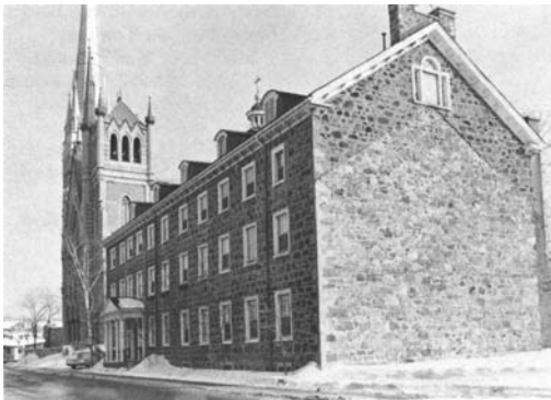
Maison Chaboillez in Longueuil, near Montreal, a former rectory and college, has been adapted as a series of ateliers and offices. (Photo by author.)
