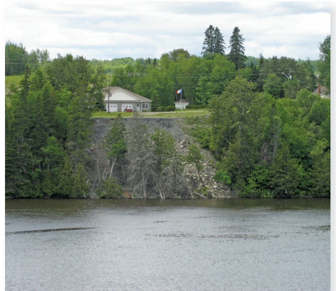
Erosion along the river bank.
