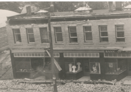
Earthquake damage to the Bank of Montreal, Port Alberni, BC, 1946.
