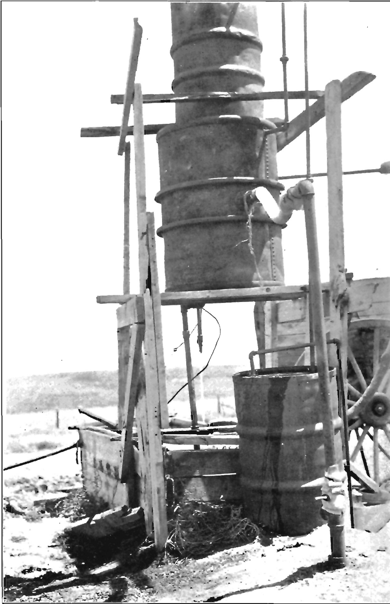
Apparatus used for saving the gas which comes with the water. Farm of John Ell. (Page 109.)
