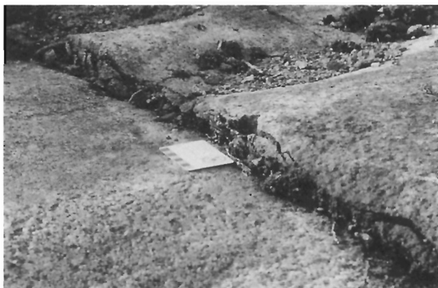
Figure 7. Neotectonic fault at Cheam View (Location 2).
