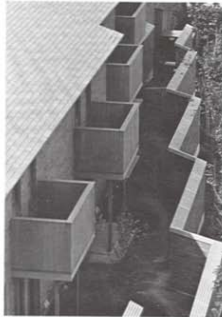
At LeBreton, a barrier wall and sound barriers on windows were used for traffic noise attenuation.
