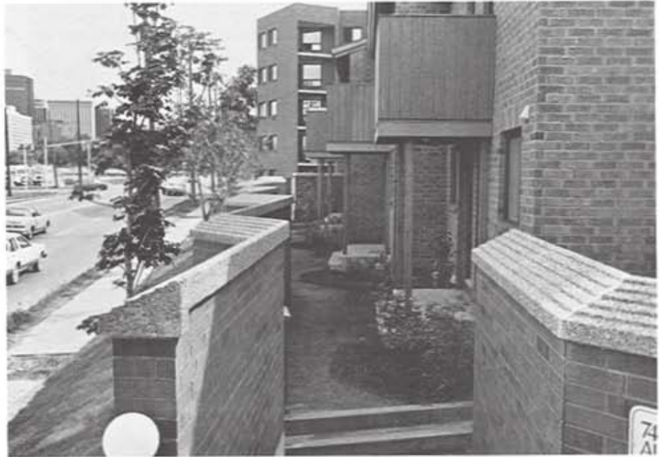
The window barrier and the roof awning for the entrance were designed as an integrated unit.
