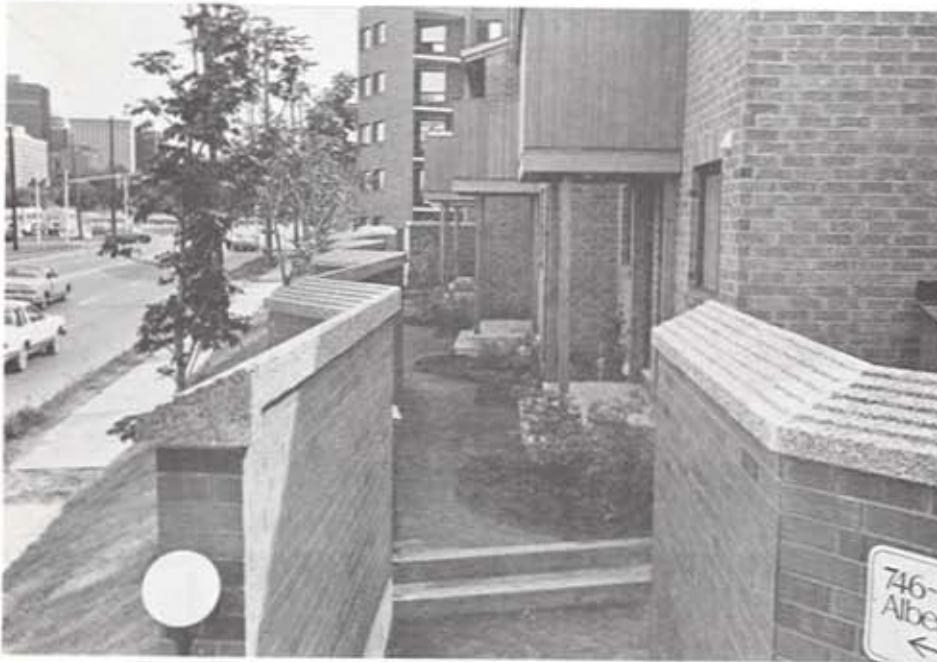
The brick wall with precast cap built along Wellington Street.
