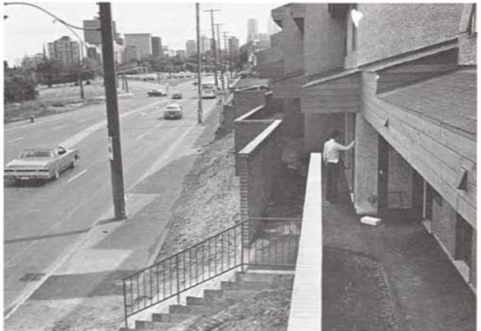
The standard brick wall used for sound attenuation at LeBreton.
