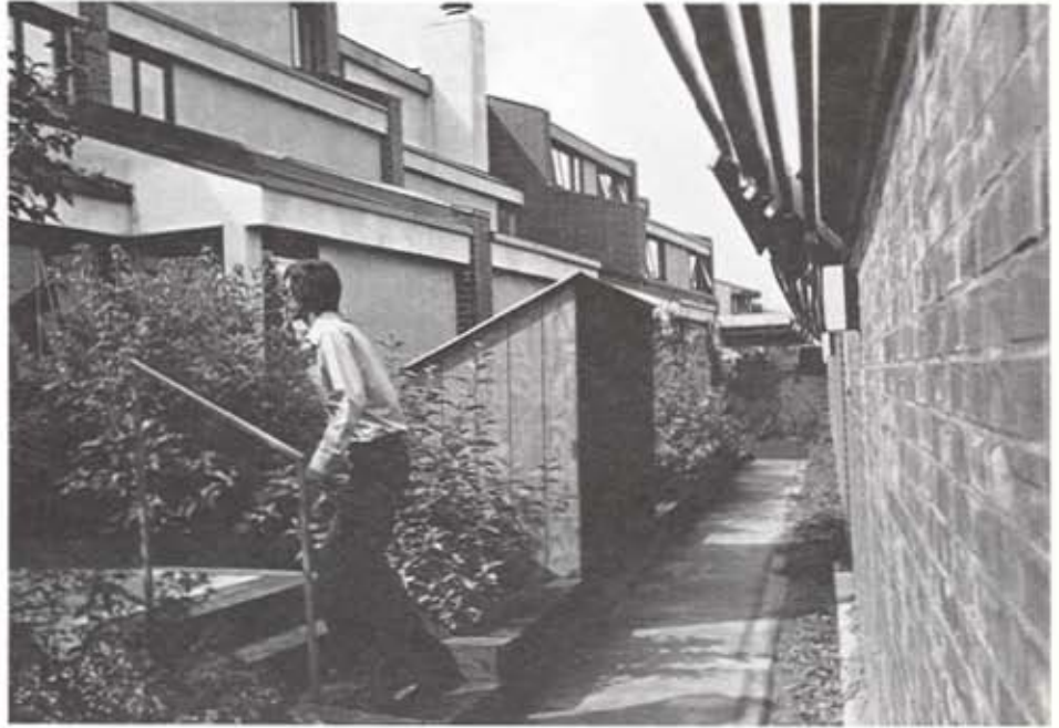
The traffic noise barrier wall was also designed to protect the entrances to the units.
