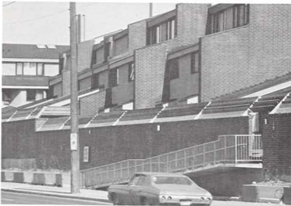
The traffic noise barrier wall of brick is topped with a louvered deflector which also reduces snow drifting behind the wall.
