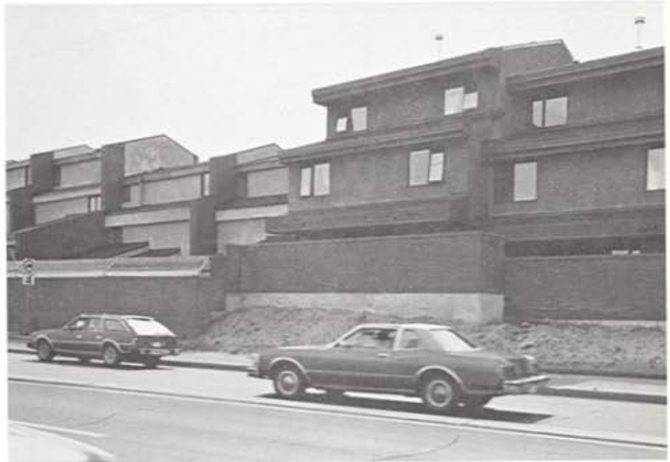
The traffic barrier walls can be designed to blend with the façades without dominating the design.
