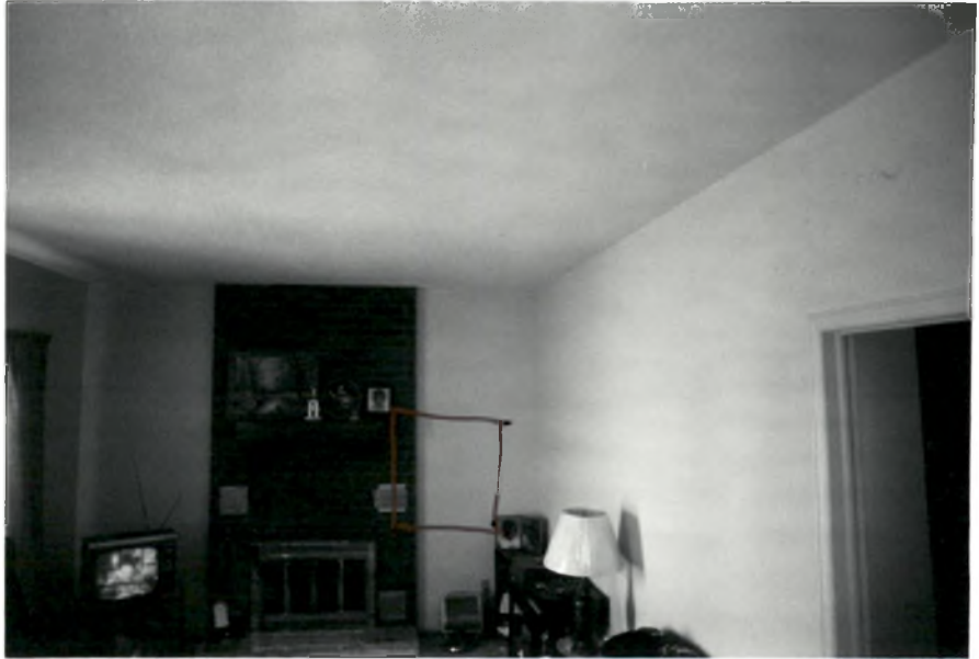
NOTE THERMOGRAM LOCATION AND PROBLEM AREA
