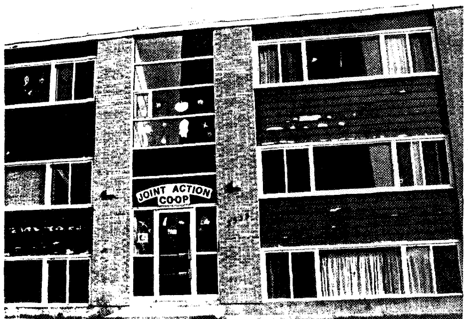
Joint Action Co-op, Regina. Lack of maintenance shows.
