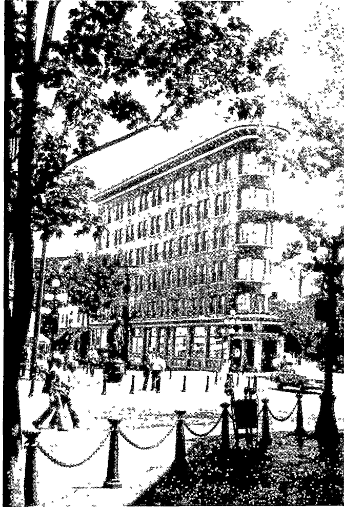
Fig.10: The Europe Hotel. A Vancouver landmark that was a market hotel that was undergoing demolition by neglect. It has been renovated and restored and is now a social housing project. Majority of units are hostels.
