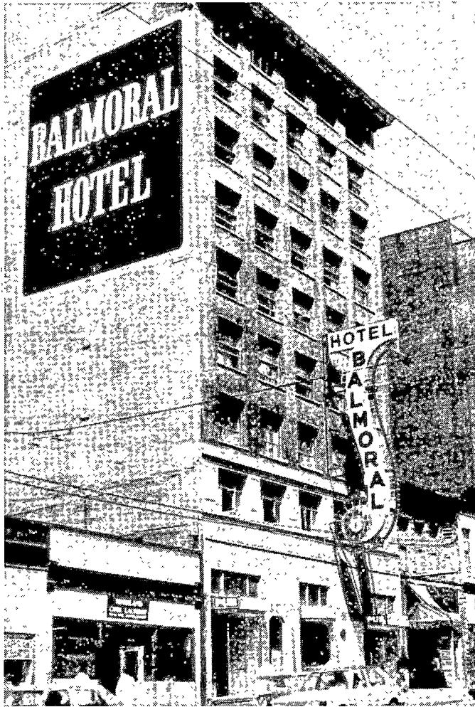
Fig.2: A typical Hotel. Pub is at grade level. (There are 27 beer parlors in study area). Laundry is conveniently located.
