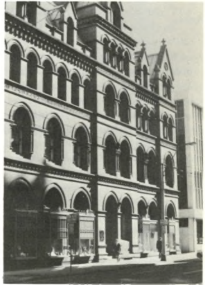
(27) THE HENRY BIRKS AND SONS BUILDING / formerly the Canada Life Assurance Building . Arch., James Balfour / 2 King Street East / 1880s. (27a) A detail of the intricate fenestration, part of the Venetian Gothic repertoire.
