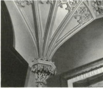
(12a) INGLEWOOD/ Arch. , William Thomas (?) 15 Inglewood Drive/c. 1855. Gothic Revival fan vaulting, interior porch.
