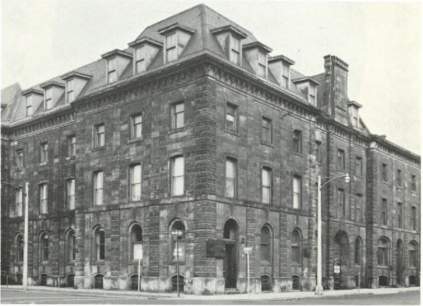
(20) COMMERCIAL BLOCK /69-73 MacNab Street North/1858. This mercantile palazzo has served the needs of Hamilton merchants for more than a century. Grimy as a Glasgow warehouse, it nevertheless reveals a master's design.
