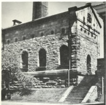
(21a) THE OLD PUMP HOUSE/900 Woodward Avenue/1859. An exterior view of Thomas C. Keefer's engineering marvel which brought Hamilton to the threshold of its prominence as a great industrial centre. Keefer was elected first President of the Canadian Institute of Civil Engineers, later to become the Engineering Institute of Canada.
