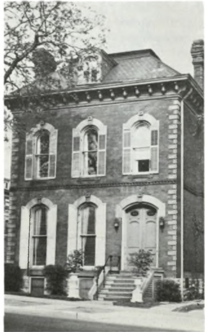
(24) 250 JAMES STREET SOUTH / Arch., James Balfour / 1870s. An instance of the popular mansard roof in its most refined form.
