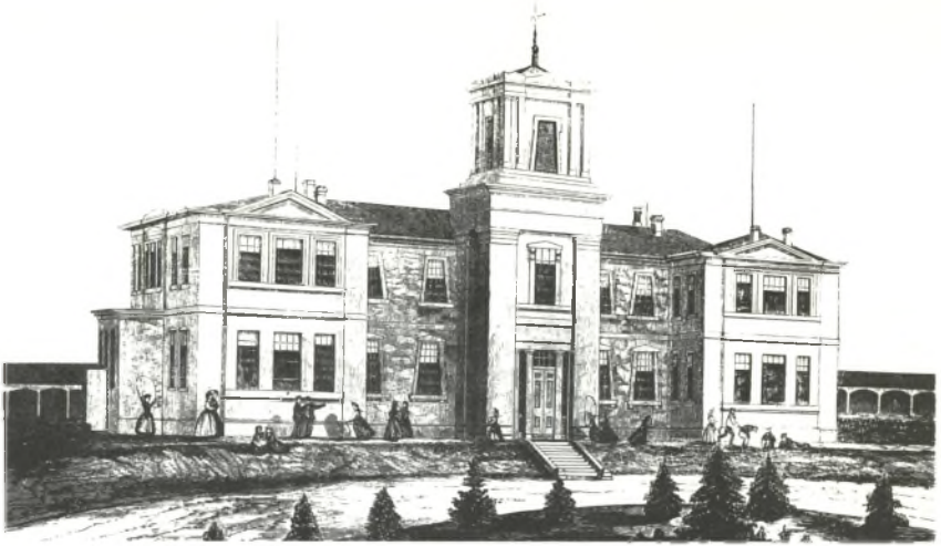
(14) CENTRAL PUBLIC SCHOOL / 75 Hunter Street West / 1853. 'The building is commodious, well ventilated, and delightfully situated, and adjacent to it are the respective playgrounds and gymnasiums for the male and female scholars . . . All drink of the same fountains of mind-invigorating knowledge, and judging from the happy faces and cleanly appearance of the whole, we should say that none have partaken in vain.' (Press notice, 1853)
