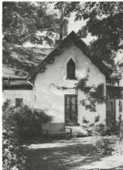
(11) GATEKEEPER'S LODGE, AUCHMAR/ 71 Claremont Drive/1855. This picturesque Gothic cottage is a reduced version of the master's house.
