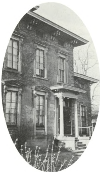
(6) 76 ARKLEDUN AVENUE/1860s. Classical Revival ornaments are here applied to an Italianate villa with distinctive overhanging roof and bracketed eaves.
