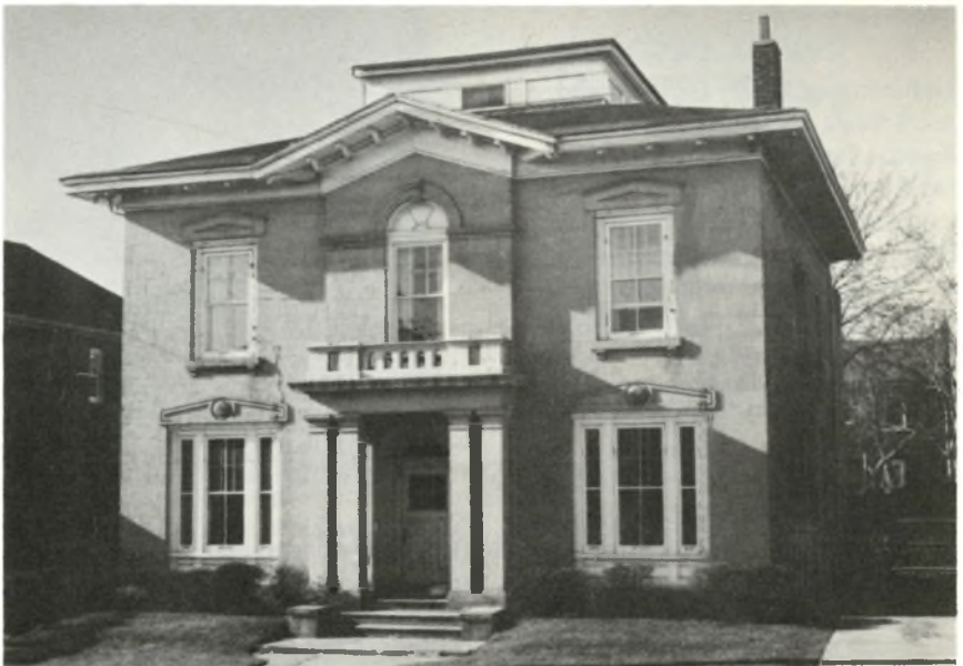
(3) THE ROACH HOUSE / 55 Barton Street West / c. 1850. Built in Hamilton limestone, this early version of the Italianate villa was designed for George Roach, a former Mayor of the City.
